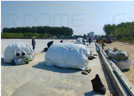
Placement of membrane units
