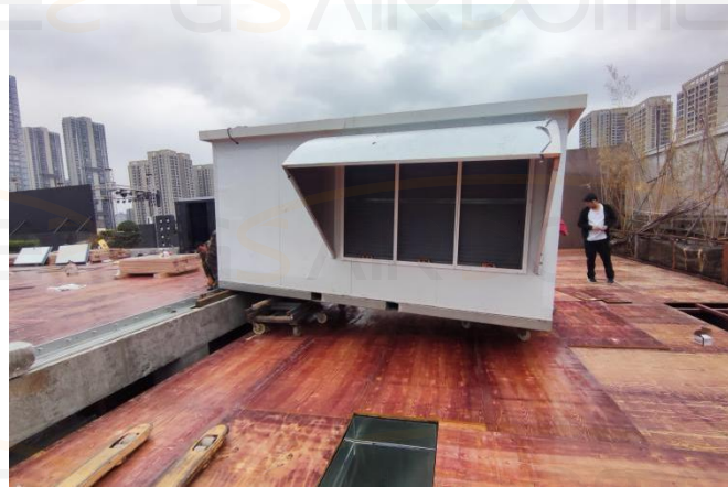
Mechanical and electrical equipment installation
