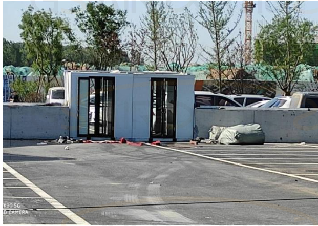
Revolving door installation
