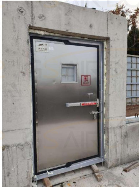
Emergency door installation
